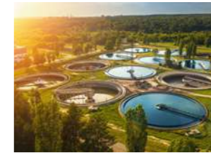
Sewage treatment plants
