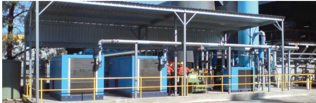
OneSteel Rod & Bar Mill Newcastle
