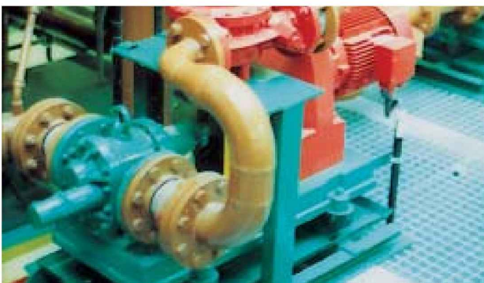
Gear pump T-GKGM in printing-ink installation
