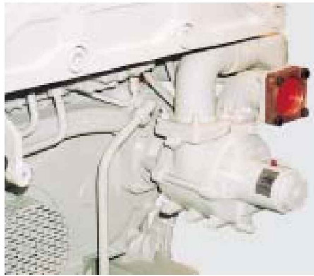
Installation of centrifugal pump KB
