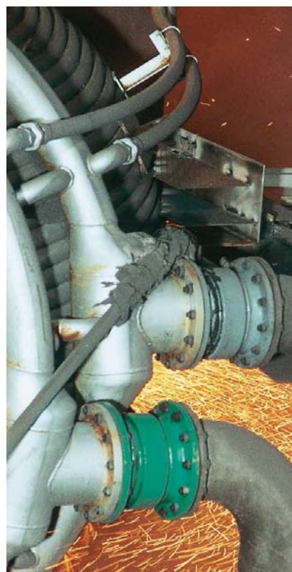
STENFLEX® Swivel Joint type DG-02L in cooling water line of exhaust pipe of furnace in a steel mill
